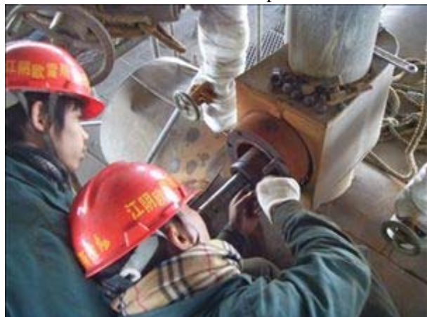
Power line valve repair
